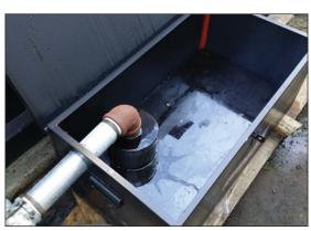
Figure 3: The tank for collecting condensate.
